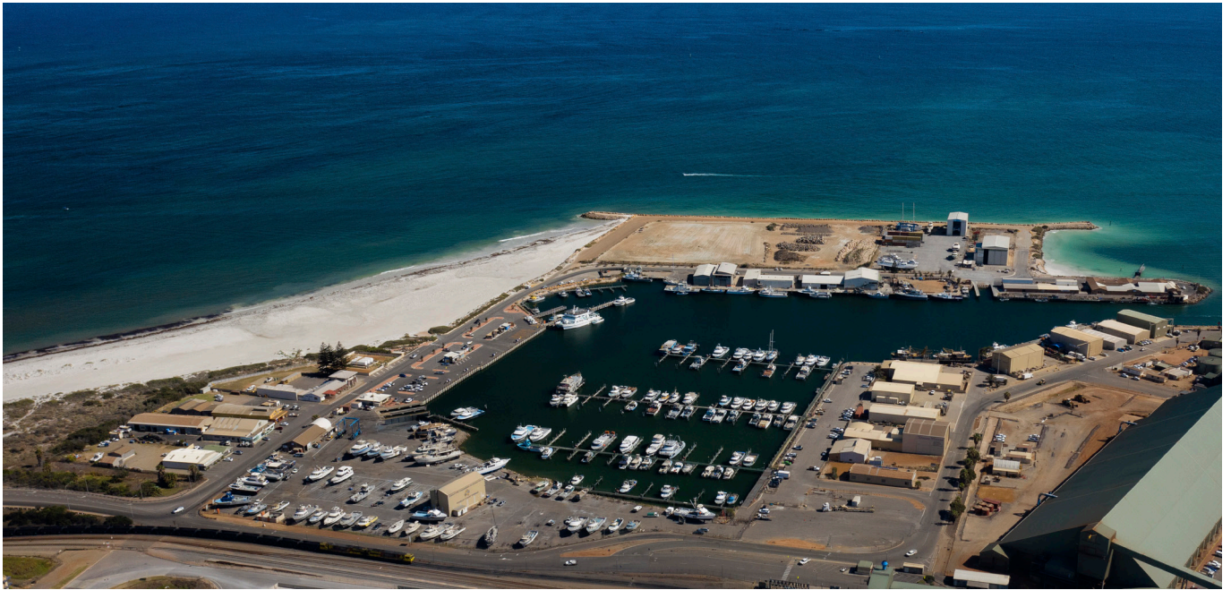
View from the south (2021)
