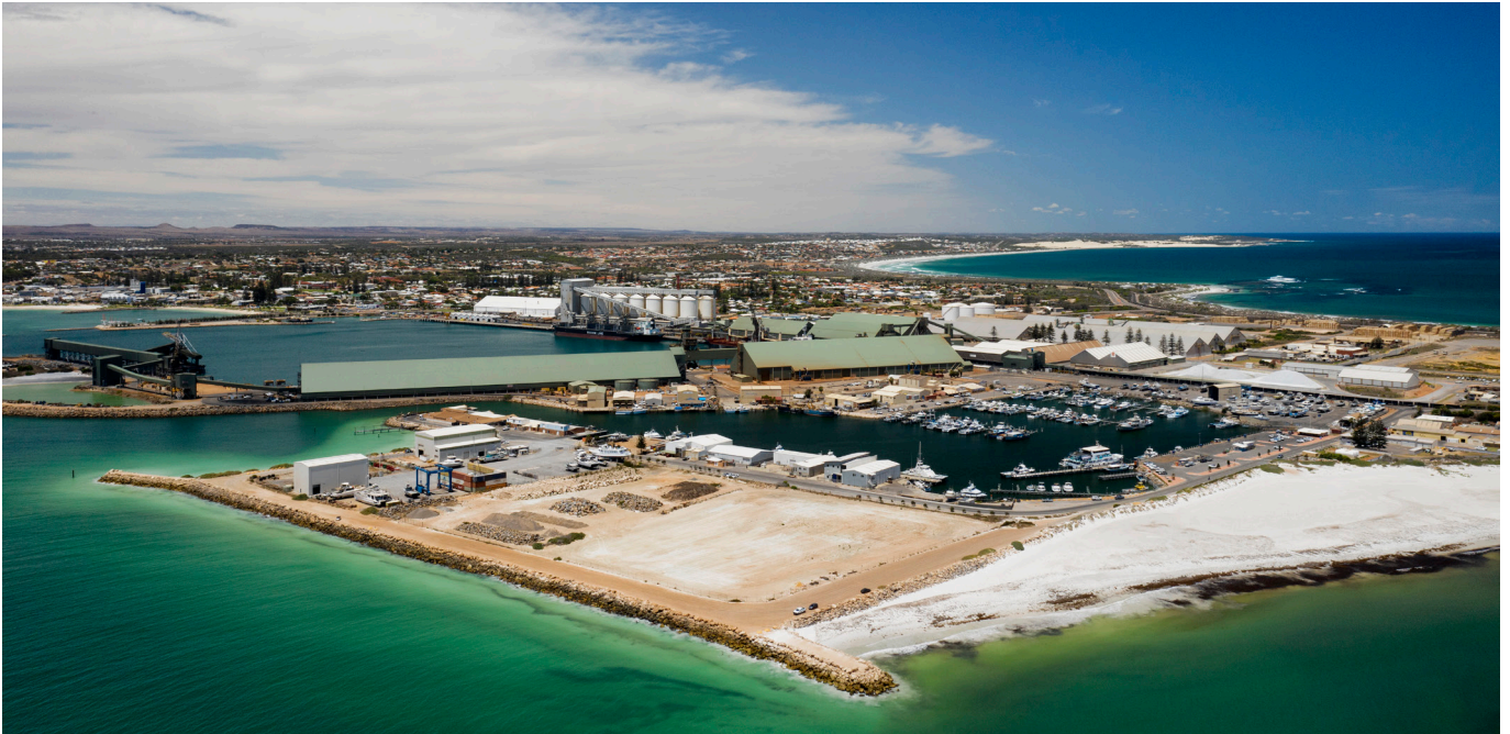
View from the north-west (2021)
