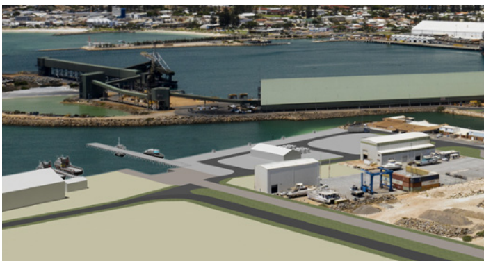
Marine Servicing and Refueling Precinct
